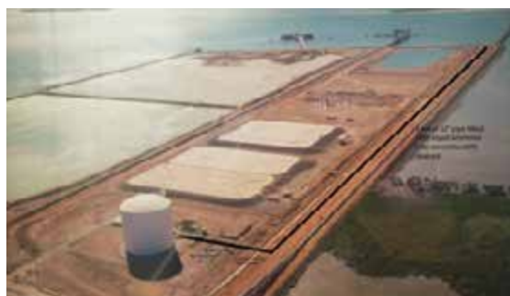
A view of the loading line with flare
