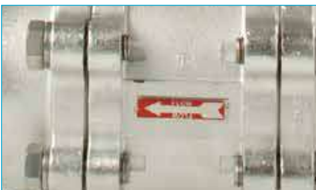
Indicator on valve body
